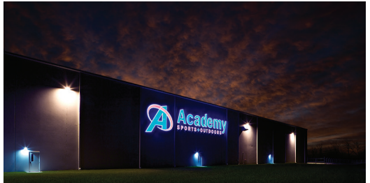
Academy Sports + Outdoors distribution center Jeffersonville, Ga. Distribution
