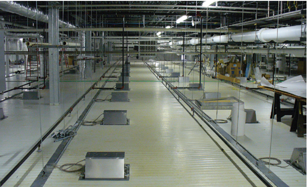
This “walkable ceiling” allows utilities and other fixtures to be more easily accessible above the plant floor, substantially reducing the risk of contamination from equipment breakdown and maintenance.
