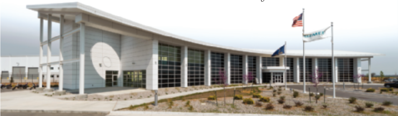
Siemens Energy, Inc. Nacelle production facility in Hutchinson, Kan.
