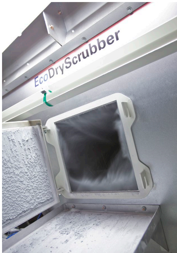
This innovative dry-scrubber system in Volkswagen Chattanooga’s paint shop significantly reduces power and heat energy use.
