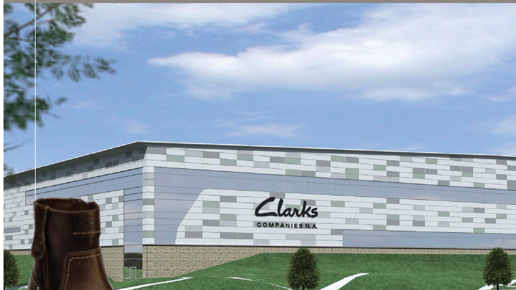
Clarks Companies, N.A. South and West Walls / Hanover, Pa.
