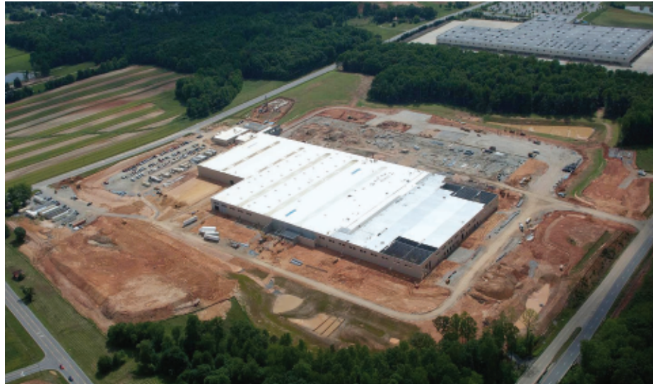
The 102-acre Caterpillar site in Winston-Salem went from groundbreaking to erecting structural steel and pre-cast panels in just four months.
